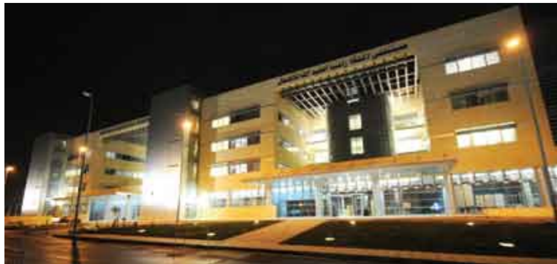
Pediatric Hospital in AL Hussein Medical City Project - Jordan
